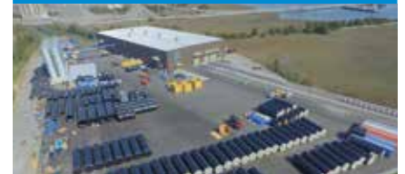
XXL PIPE PRODUCTION FACILI- TY CHARLESTON, SC/USA
