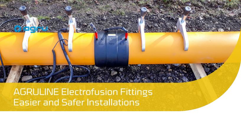
In addition to its HDPE butt fusion fittings, AGRULINE includes a line of electrofusion fittings made with PE 100-RC. This modern resin allows AGRU to produce the highest quality electrofusion fittings on the market. In a comprehensive series of tests, the renowned HESSEL Ingenieurtechnik GmbH test institute showed that the service life of AGRU's PE 100-RC E-couplers is about 10 times longer than standard E-couplers currently available on the market under test conditions (Figure 1).
