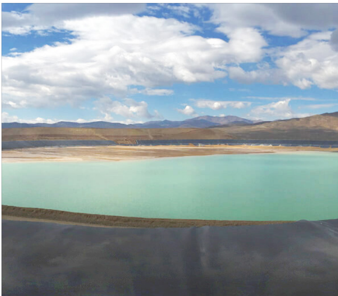
Double-Lined Solution Ponds
