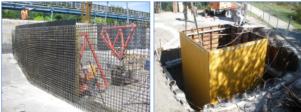
(Examples: Assembly of AGRU CPL onto wooden formwork – cast in situ applications)
