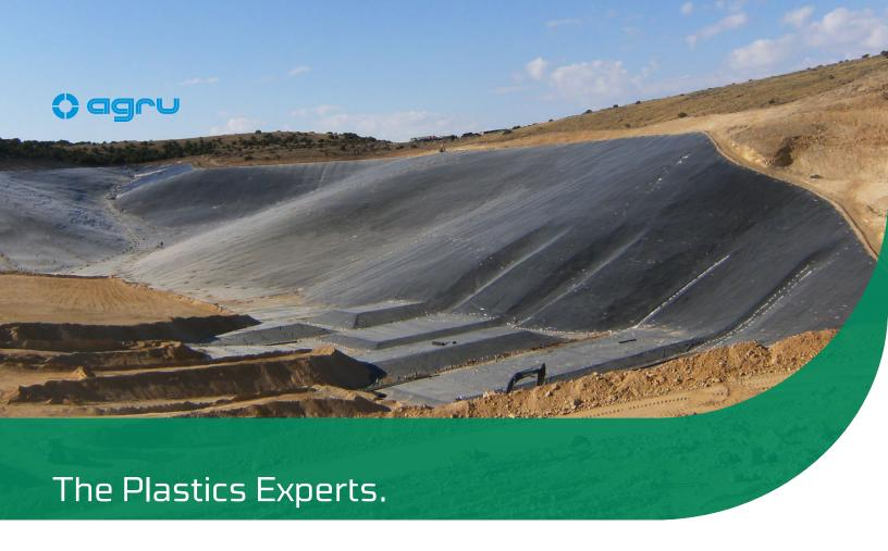
AGRU geosynthetic liners are manufactured with only the highest-grade polyethylene resins using the calendared flat-die extrusion process. This manufacturing technique allows for coextruded liners with multiple features such as surface textures and secondary properties. The benefit of this process is liner with consistent textures, stud and spike heights, thickness, and an array of secondary features without compromising liner integrity.
