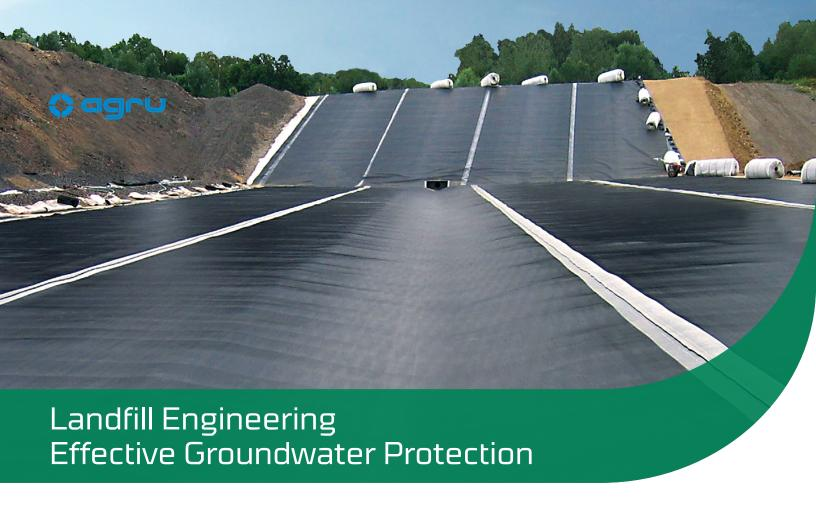
Landfill lining systems are chosen depending on the materials expected to be stored on site. In some cases, a second layer of HDPE or LLDPE geomembranes is installed alongside other geosynthetics. In every case, however, the geomembrane is always the primary lining element at a landfill to prevent rainwater penetration when the surface of the cell is being lined, and to prevent groundwater from being contaminated via the landfill cell's base liner.
