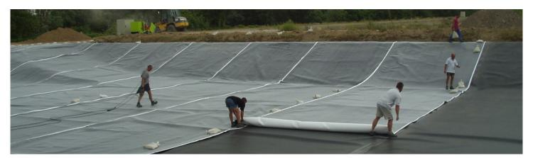
HDPE geomembranes act as a seal for central ground filters that collect rain water from flight operation areas with contamination from surface de-icing.
