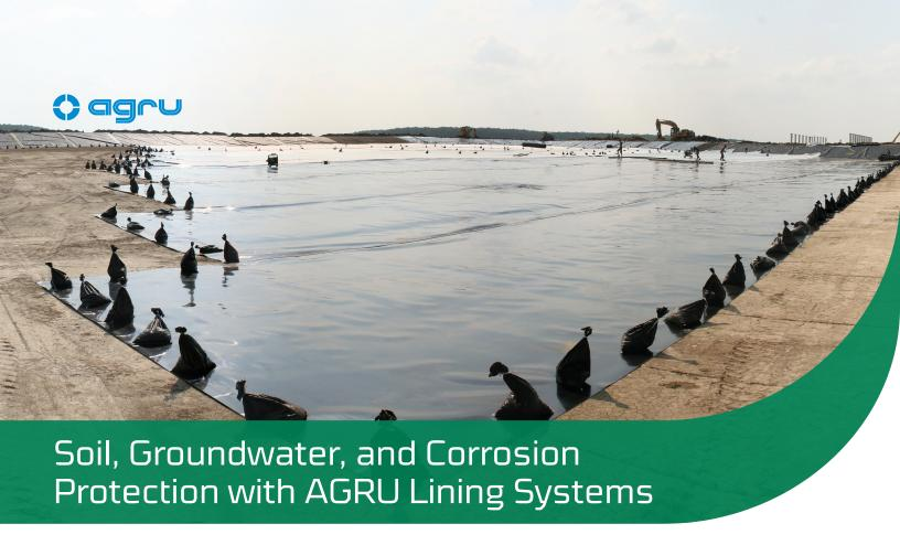
AGRU Lining Systems are suitable for virtually any application. Chemical-, root-, rodent-, and UV-resistant, these tear-proof and extensible geomembranes are designed to last a long time.
