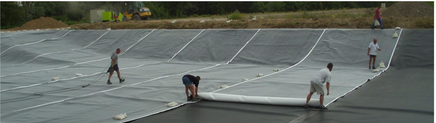
HDPE geomembranes act as a seal for central ground filters that collect rain water from flight operation areas with contamination from surface de-icing.
