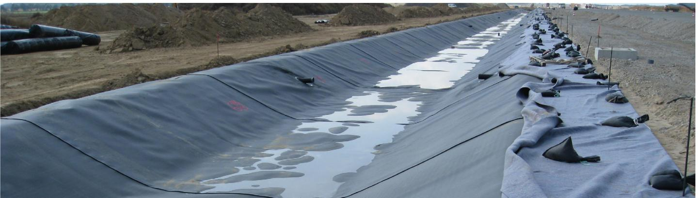
Local ground filters are also being made from HDPE geomembranes to go next to the runways and taxiways. These are being used to treat rainwater with impurities from flight operations and surface de-icing before it is transferred to the central ground filters.
