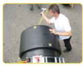
When installing the coupling, taking care that the coupler's connectors and that the preheating code as well as the welding code are is easily accessible. The assembly can be assisted by evenly distributed blows with a soft hammer until the marked insertion length (marked
