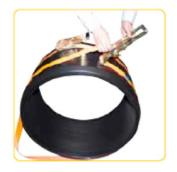
Both tension belts must be put into the groove and tightened as follows.
