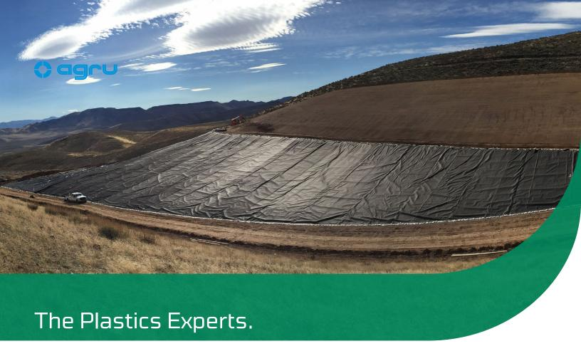
AGRU America's structured geomembranes are manufactured on state-of-the-art manufacturing equipment using the flat die calender manufacturing process, a method that produces a more consistent core thickness and greater physical properties than other processes, such as the blown film extrusion process. AGRU uses only the highest-grade HDPE and LLDPE resins manufactured in North America.
