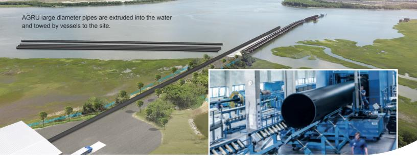
For high volume flow applications, AGRU provides a large diameter piping system up to OD 2500 mm (98.4 in.) made from PE100, PE100-RC or PE4710 resins. The better long-term hydraulic properties, which save operation costs, are based on a high resistance to corrosion, wear and tear and UV radiation. These properties, together with the system's fast and efficient installation, make AGRULINE large diameter pipes the perfect solution for both on- and offshore projects.
