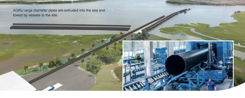
For high volume flow applications, AGRU provides a large diameter piping system up to OD 2500 mm (98.4 in) made from PE100, PE100-RC or PE4710. The better long-term hydraulic properties, which save operation costs, are based on a high resistance to corrosion, wear and tear and UV radiation. Together with its fast and efficient installation, this is the perfect system both on- and offshore.
