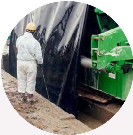
Downfeed of the panel using a drum with an electric drive unit.
