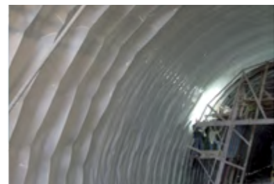
Hot Weld Joint In Tub Construction
