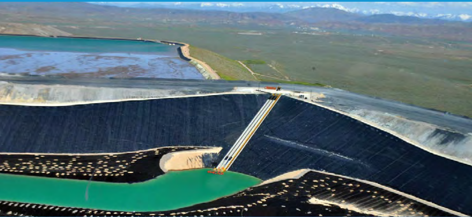
Figure 3: Agru America Mining Installation
