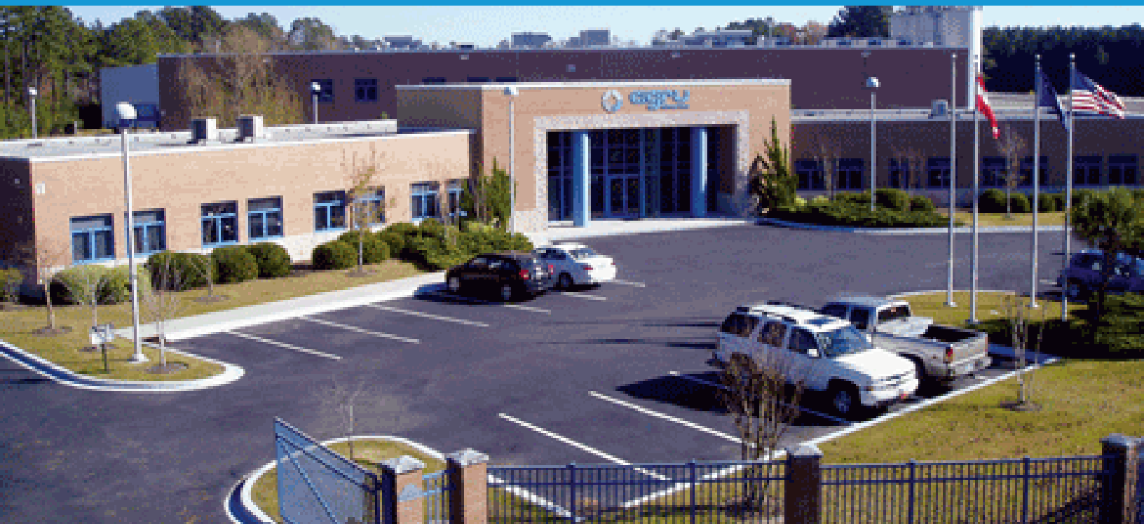
Figure 1: Georgetown, SC Agru America Headquarters and Production Facility
