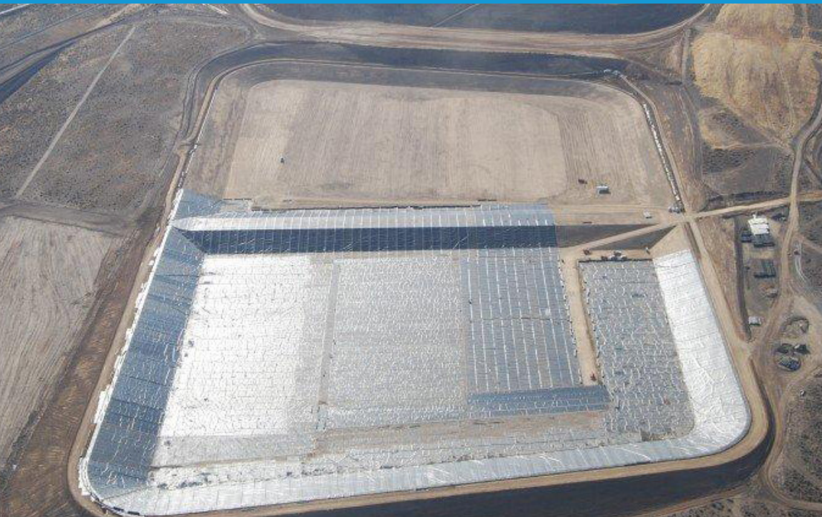
Figure 1: Installation of Drain Liner® as secondary Geomembrane on project in Utah
