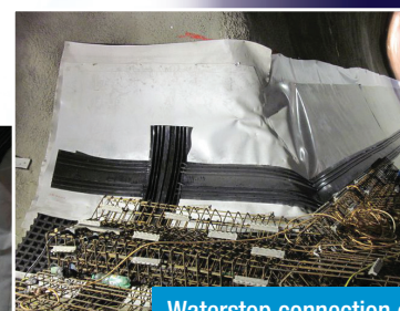
Waterstop connection of main tunnel and crossway
