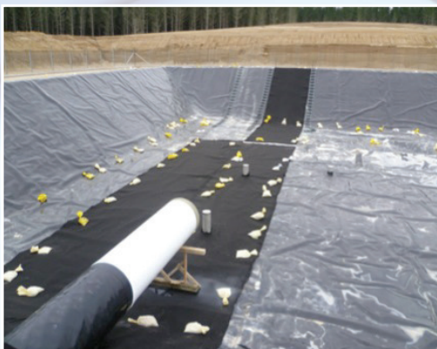
Drainage Composite on top of Primary HDPE Liner
