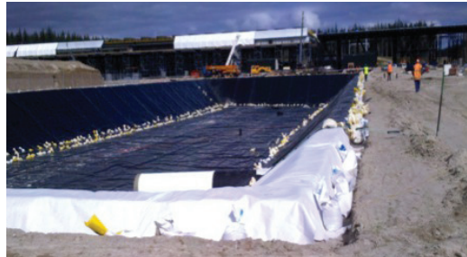
Primary Layer: AGRU HDPE Liner with nonwoven Geotextile 300g underneath
