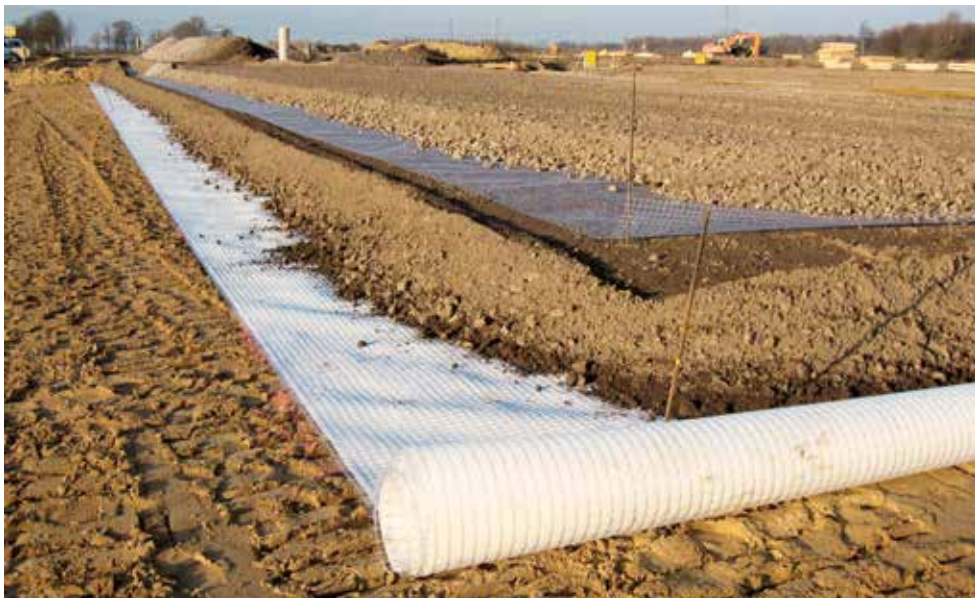
Similar to geotextiles, geogrids offer soil and waste mass stabilization solutions that can be of critical importance in CCR management and containment facilities.
