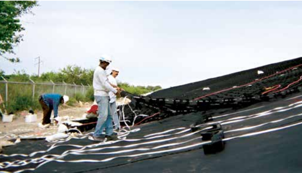
Geotextile applications include filtration, separation, stabilization, dewatering, cushioning, and erosion control, all of which can play critical roles in CCR containment and management.
