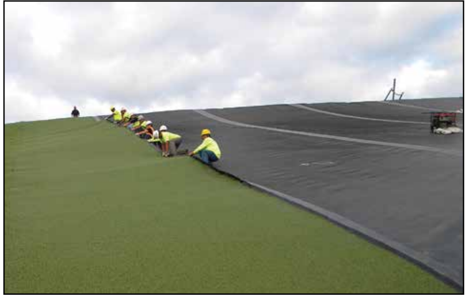
After the geomembrane is placed, the engineered turf is quickly and easily installed by simply sewing roll edges together and laying it on top of the underlying geomembrane for instant aesthetic appeal.
