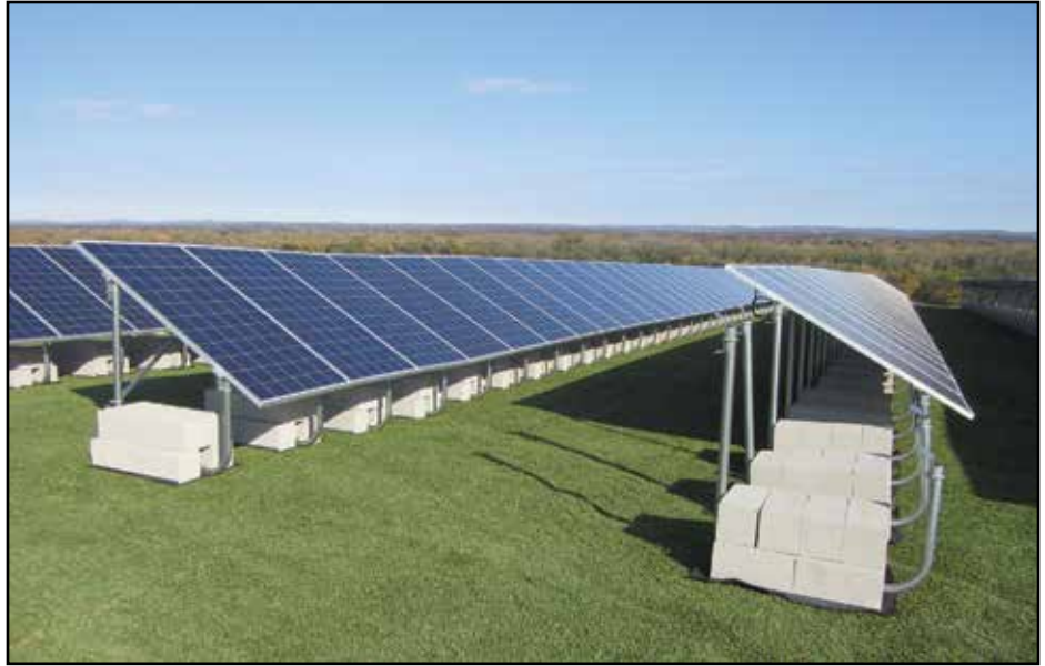
PV solar arrays panels being installed and ballasted on the System without the need for any penetrations into the cap.
