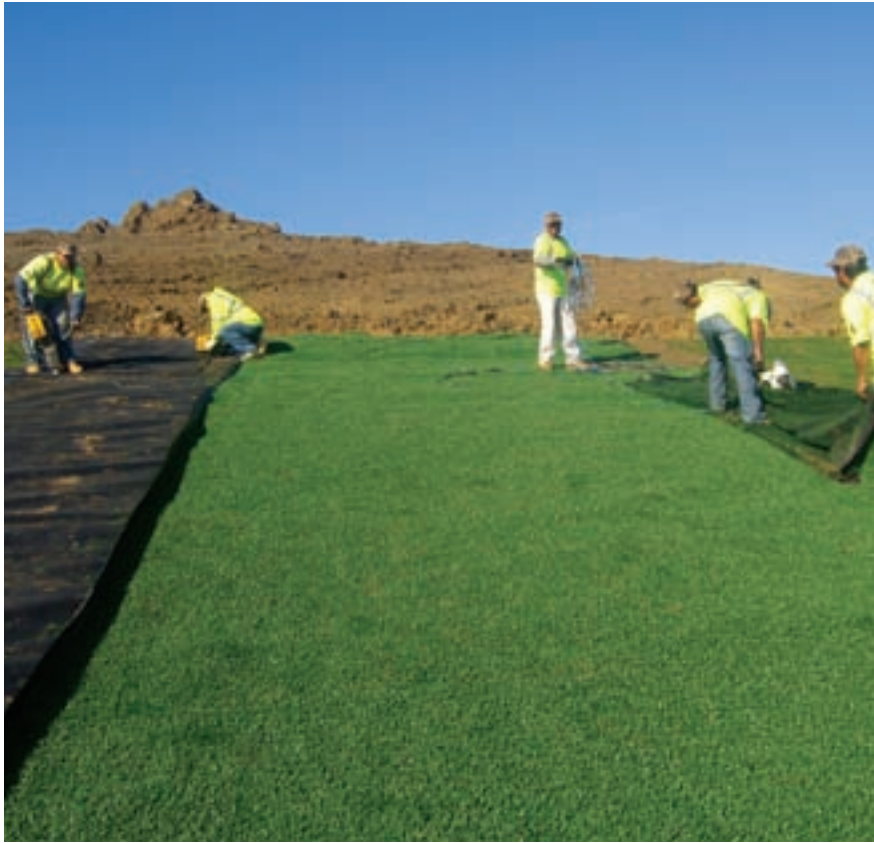
Figure 4 | The synthetic turf system at the LaSalle-Grant Landfill proved cost-effective, relatively efficient to install, and it controls fugitive emissions, erosion, leachate, and siltation.
