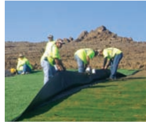
Figure 4 | The synthetic turf system at the LaSalle-Grant Landfill proved cost-effective, relatively efficient to install, and it controls fugitive emissions, erosion, leachate, and siltation.
